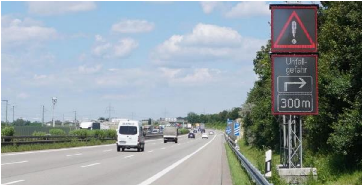
Figure 25: Example for a system, warning drivers entering a rest area or parking site (Die Autobahn 2024)
